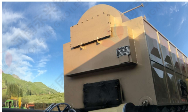
2018.05.07 固始县金达木业有限公司2吨手烧生物质蒸汽锅炉 2018.05.07 2t/h DZH manually feeding biomass boiler in Henan Jinda Wood Industry Co.,Ltd
