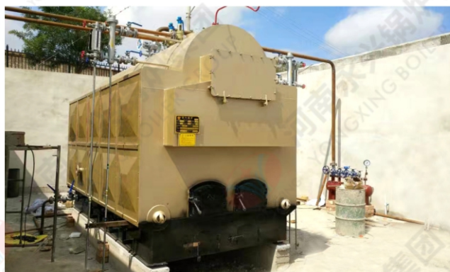
2013.09 新疆顺河天一纺织厂2吨手烧生物质锅炉 2013.09 2t/h manually feeding biomass boiler in Xinjiang Tianyi textile factory
