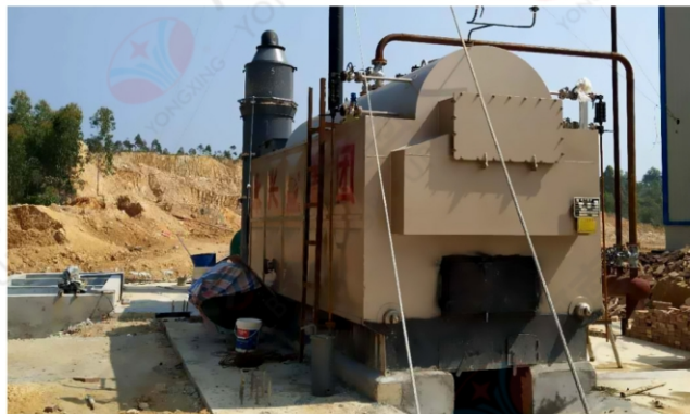
2018.04.28 湖北永光化工有限公司2吨生物质蒸汽锅炉 2018.04.28 2t/h DZH manually feeding biomass boiler in Hubei Yongguang Chemical industry co.,ltd
